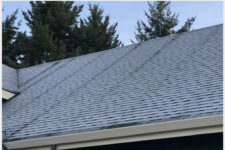
IMAGE 1.2: SIP ROOF WITH I-JOIST SPLINES
