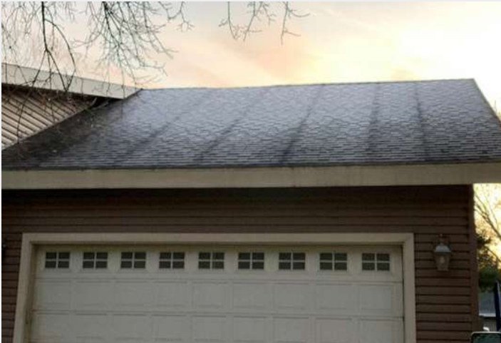
IMAGE 1.3: SIP GARAGE ROOF
