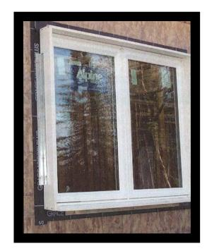
Figure 12. Alternate Window Box Mount
