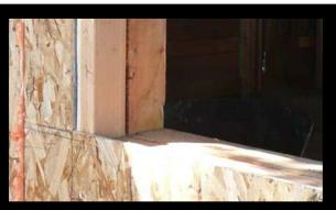
Figure 7. Retrofit Panel Routed for Window Box
