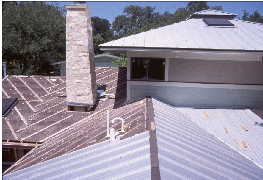
Figure 6: Diagonal furring strips under metal roofing
