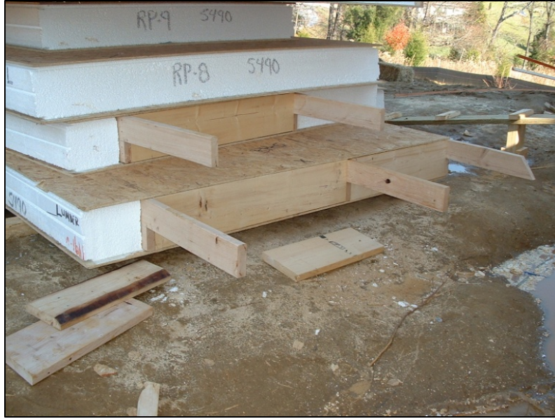
Figure 4: Embedded rafter tails
