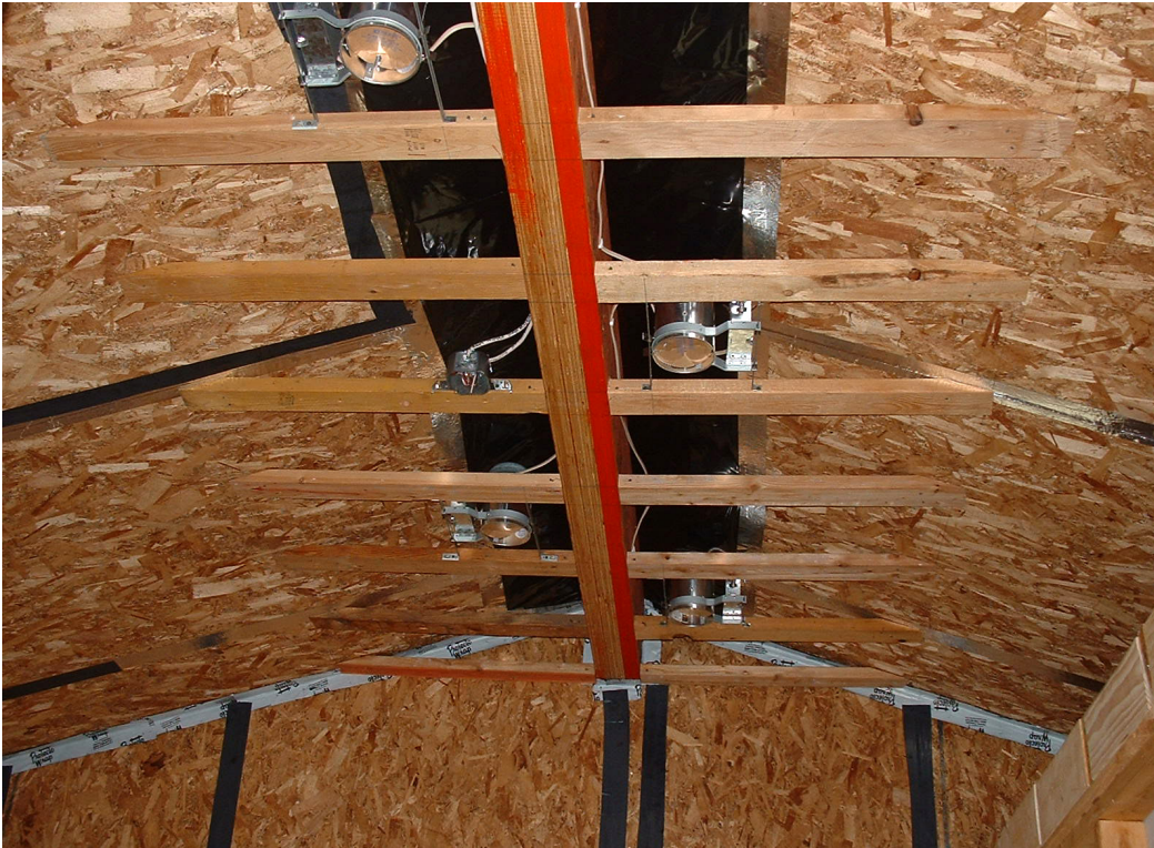
IMAGE 9.8 FURRED-DOWN CEILING FOR CAN LIGHTS
