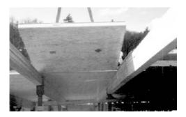
Upon receiving your roof panels, count them and check the sizes. In most cases roof panels are not fabricated at the factory because roofs tend to vary from the shop drawings. If they have been factory fabricated, double check for accuracy. Also, check the edge treatment. You may have to plane your lumber or I-joists to fit the recesses. If the panels aren't being installed immediately, cover the panels and lumber until ready for installation.
