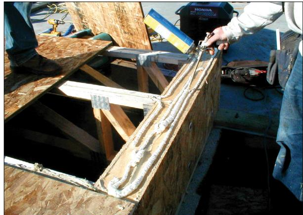
Proper sealing is especially important when installing SIP roofs. The ridge of a SIP roof can use either bevel-cut SIPs for a flush joint or a beveled foam block insert. The ridge detail is a critical construction detail that requires attention to sealing using methods as noted above. Manufacturer specifications will provide specific sealing details designed to prevent moisture movement.
