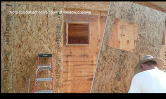
**Figure 8. Window Box with Retrofit Panel**
