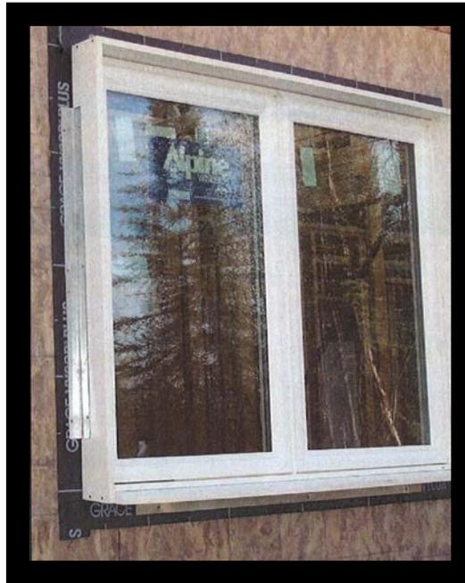
**Figure 12. Alternate Window Box Mount**
