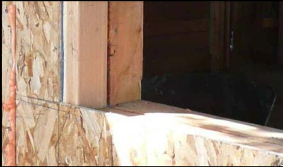
**Figure 7. Retrofit Panel Routed for Window Box**
