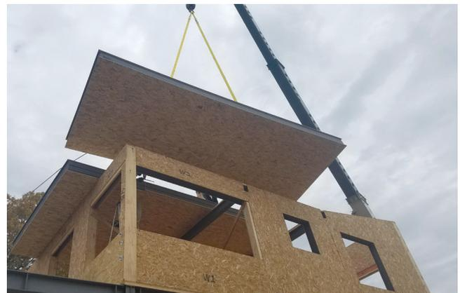
However, dimensional lumber is used in conjunction with SIPs for some specific connection details. For example, solid chord members using 2x dimensional lumber are required at each end of each SIP shear wall segment. For SIPs used as horizontal diaphragms subjected to wind or seismic loading, a 2x dimensional lumber boundary member is used.
