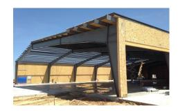
Flat Iron, CO: Originally designed with 10" Roof SIPS, using PREMIER GPS SIPS, the project was able to convert to 8" Roof SIPs. The thinner roof SIPs met all code requirements and eliminated the need for an additional two truckloads of SIPs.
