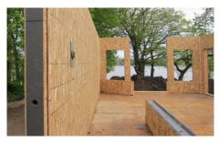
Lakeside Residence, MN: Large Premier GPS SIPS feature a solid insulation core to eliminate thermal breaks, and create a structure 15 times more airtight and 40-60% more energy efficient than stick framing methods.
